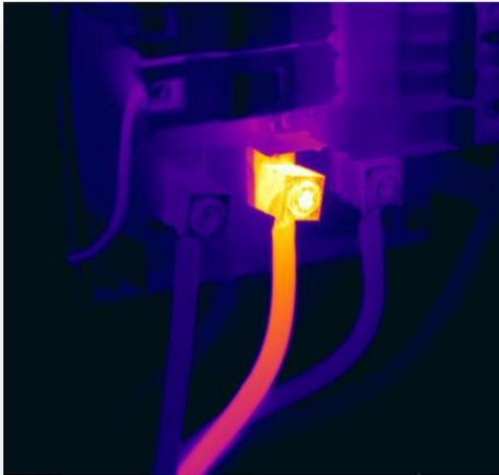
**Infratech** Electrical Infrared Inspections are performed while the Electrical system is under load, preventing shutdowns while the procedure is being completed. Inspections will allow maintenance personnel to allocate labour, time and materials for efficient shutdown repairs. High volumes of electrical equipment can be inspected in a short period of time with an extremely high degree of accuracy.
